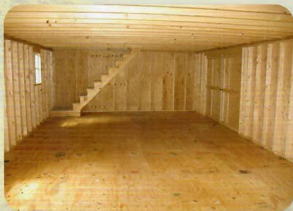
Showing the interior of the 2 Story
